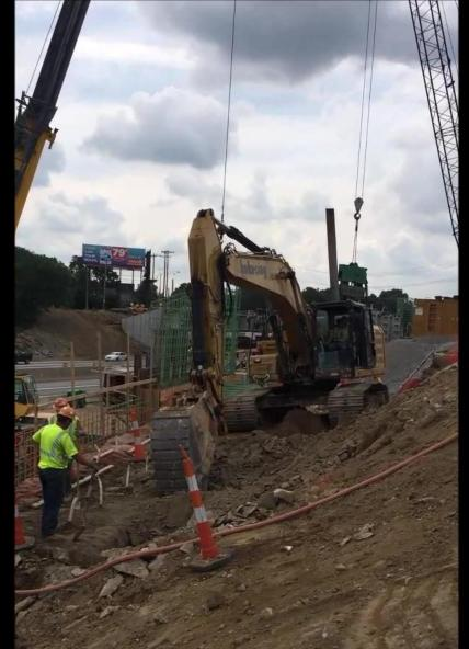
Removing Surface of Jet Grout Soilcrete Cleveland, Ohio, 2018
